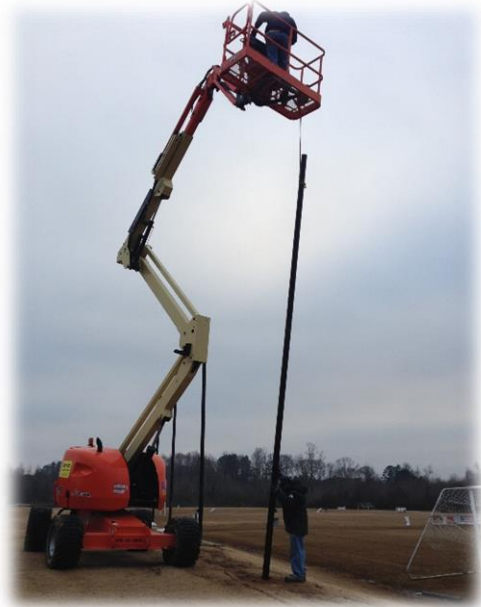
We designed and installed backstop netting with metal poles and 4 inch mesh net behind all 12 of the big goals.
